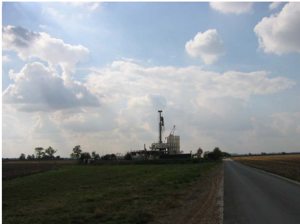
Photograph No 1 – Drilling Rig on site at Cold Hanworth, Lincolnshire
