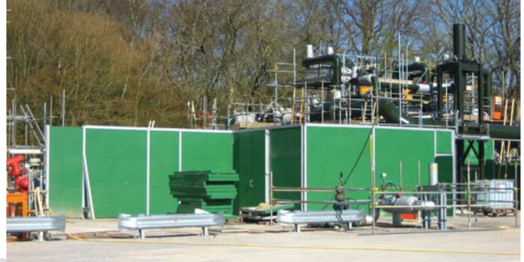
Typical acoustic fence
